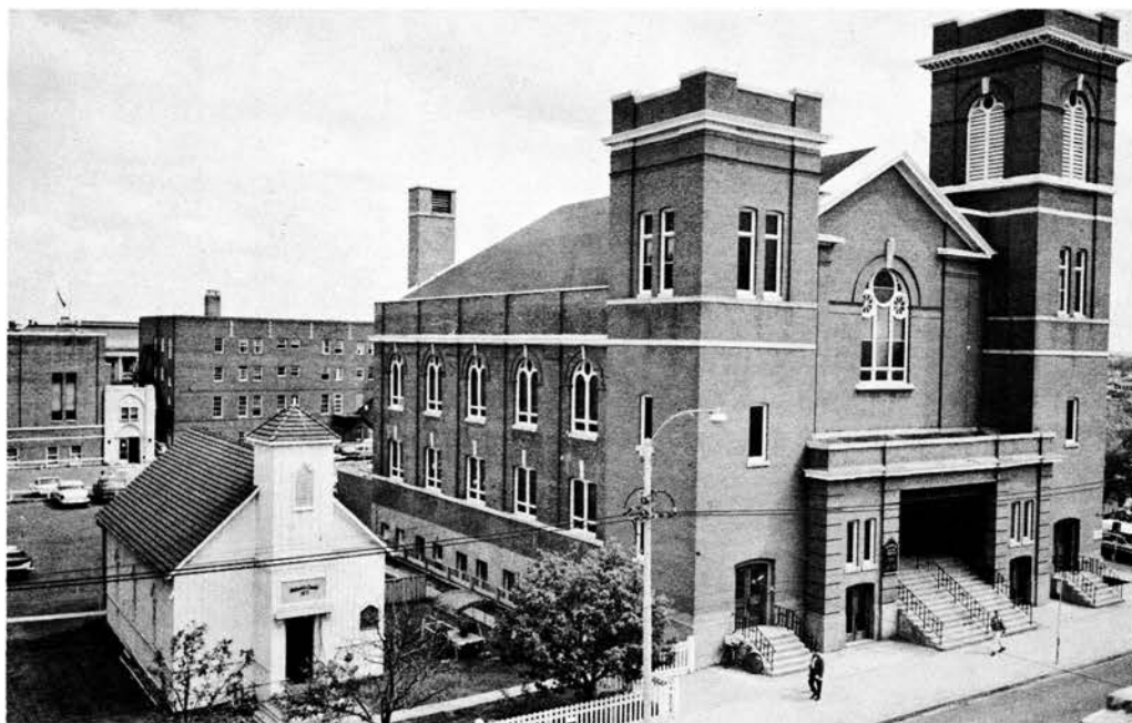
Tiny original George McDougall Church, over 100 years old, beside modern McDougall United Church in downtown Edmonton.
