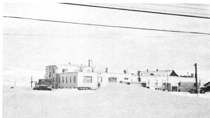
Maynard McDougall Memorial Hospital in Nome, Alaska
