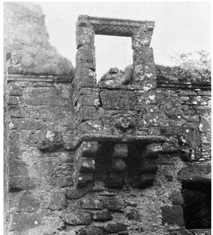
Oriel window - north wall of Gylen. Photo by W. M. Macdougall.
